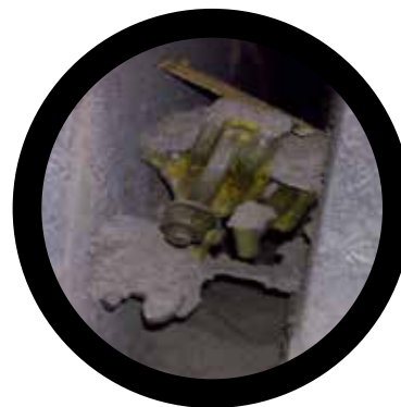
Spot the scaffolding clamp!
