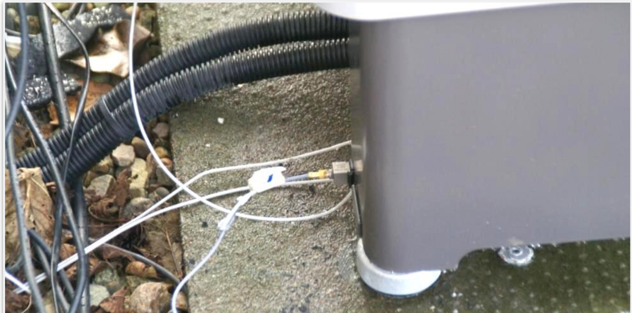
Picture 5-13. 422 Fraserburgh (Replacement), Casing-mounted Accelerometer
