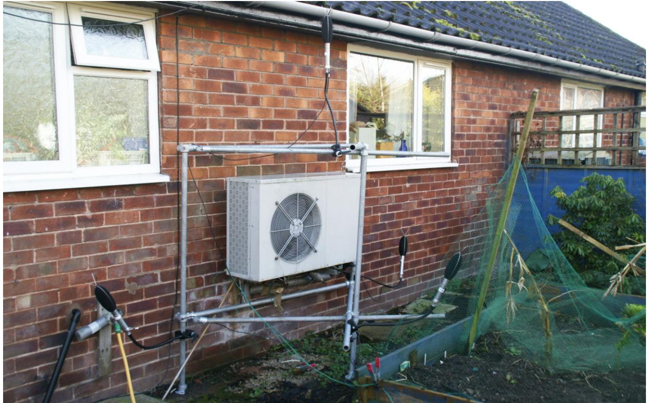
Picture 5-15. 443 Cheshire West, ASHP and Microphone Arrangement
