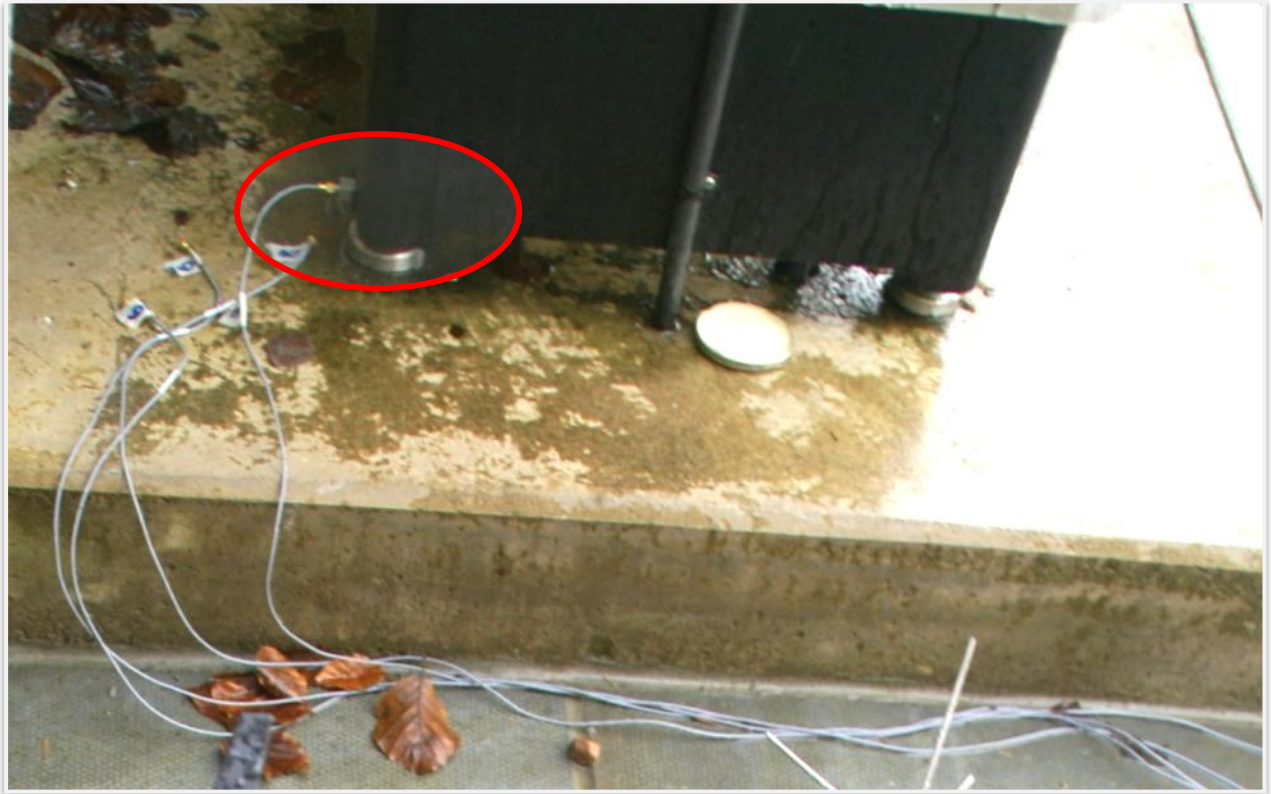
Picture 5-8. 418 Central Buchan, Casing-mounted Accelerometer
