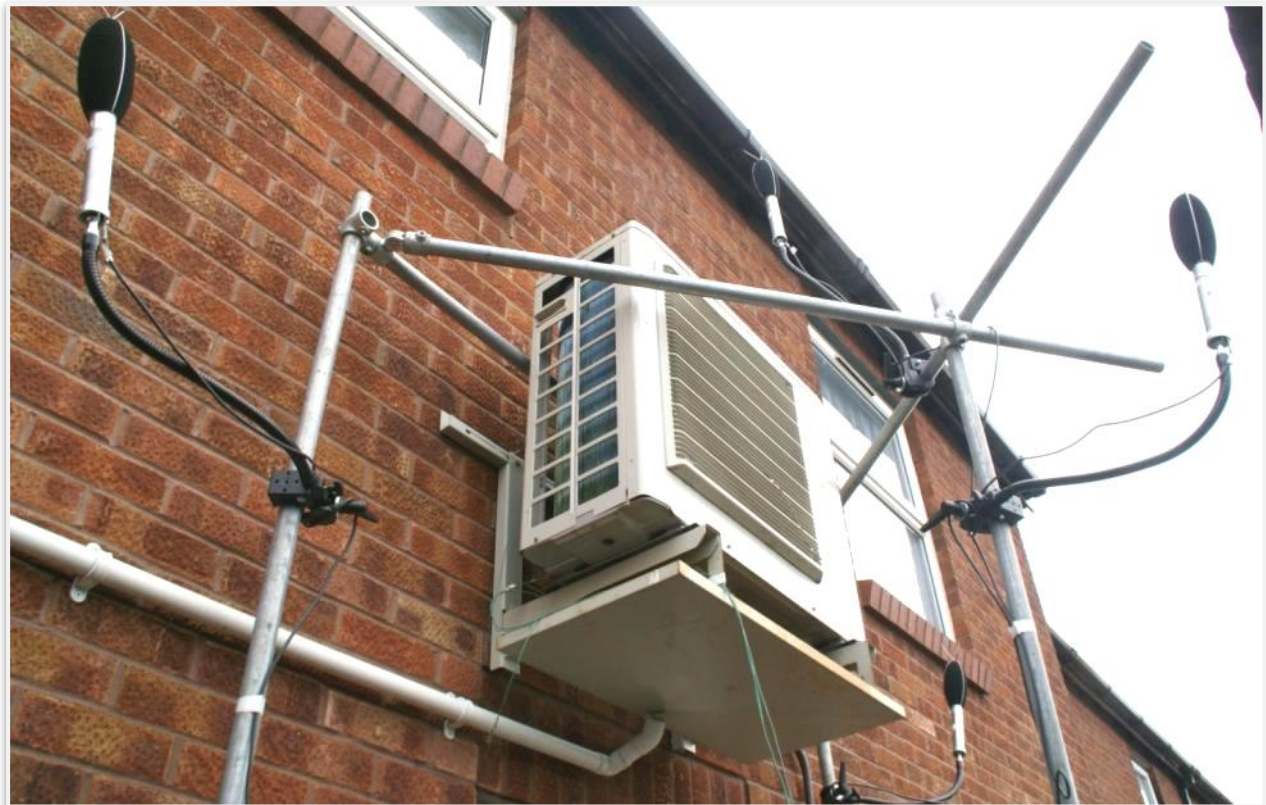
Picture 5-4. 486 Stroud, ASHP and Microphone Arrangement
